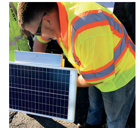
Connect batteries and test components before erecting the pole system.
