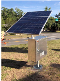
Connect batteries and test components before erecting the pole system.
