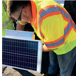
Connect batteries and test components before erecting the pole system.
